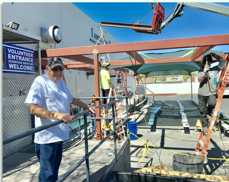
Ted Dunne overseeing the new awning install.
