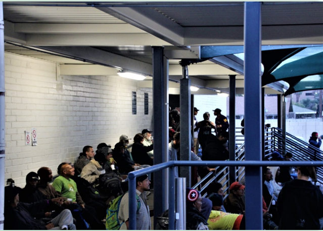
completed awning and safety railings providing outside guests safe shelter
